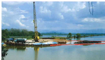
Containment of sediment for earthwork filling
