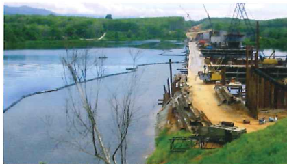
Bridge construction containment control
